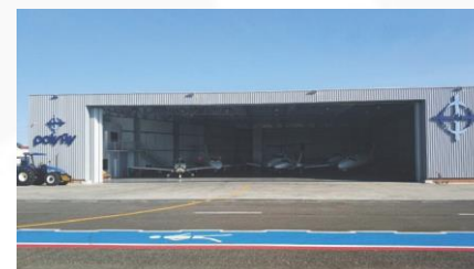
Navegantes, SC – Brazil Hangar PolyFly
