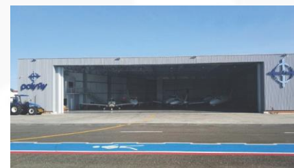
Navegantes, SC – Brazil Hangar PolyFly
