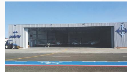
Navegantes, SC – Brazil Hangar PolyFly
