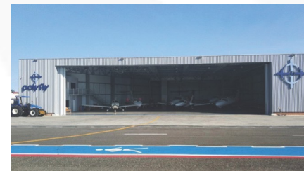
Navegantes, SC – Brazil Hangar PolyFly
