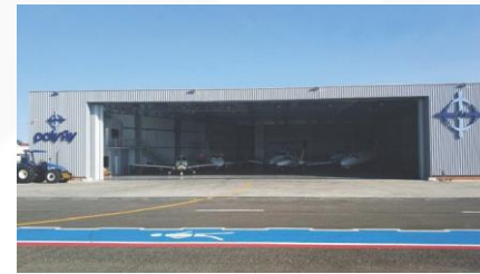
Navegantes, SC – Brazil Hangar PolyFly
