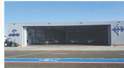
Navegantes, SC – Brazil Hangar PolyFly
