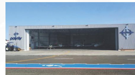
Navegantes, SC – Brazil Hangar PolyFly
